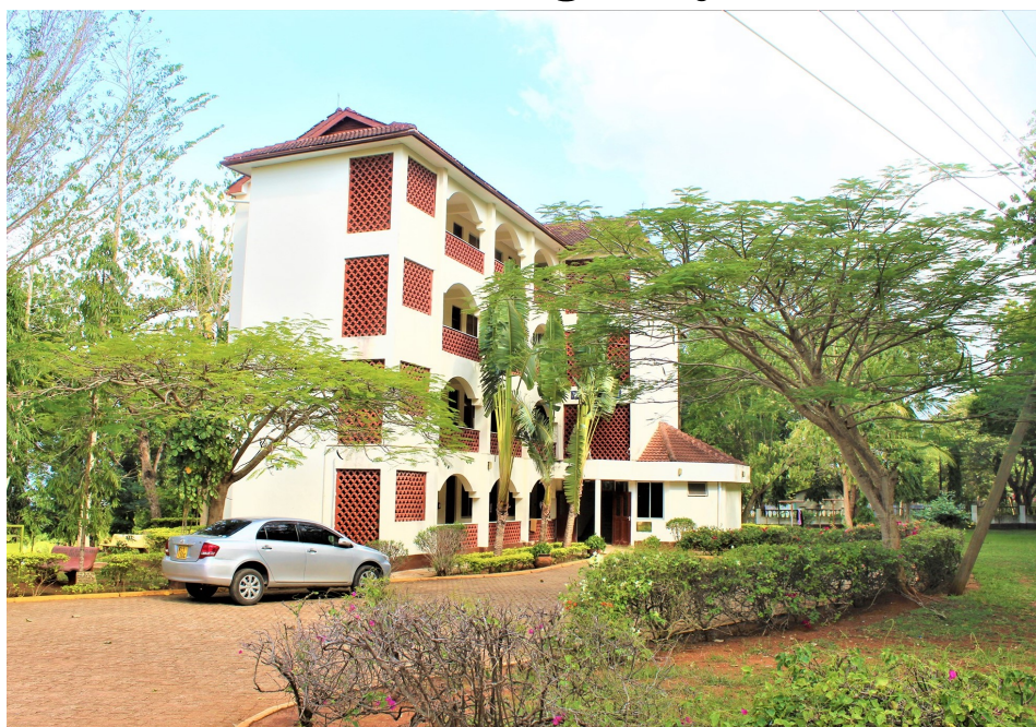
A section of the hostels at the Matuga Campus.
